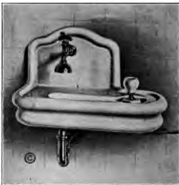
FIG. 36.— Wash-hand basin, with sanitary bubbling cup at the right, which flows when the lever below is pressed down. (American Medical Association Building.)
